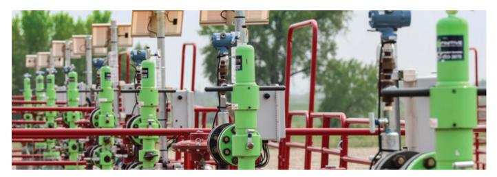
Figure 8: An example of Bayswater utilizing solar arrays to help power wellheads on a Colorado production site.
