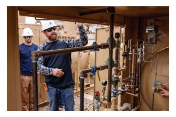
Figure 9: A Bayswater employee showcasing the instrument air pneumatic devices on a Colorado production site.
