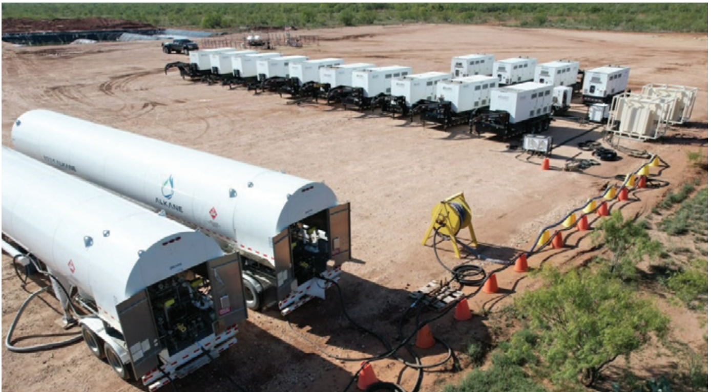
Figure 19: An example of power generation on a Texas Bayswater location utilizing LNG as the fuel source.
